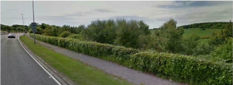
FIG 3 Existing woodland and hedging along A92 Road.
